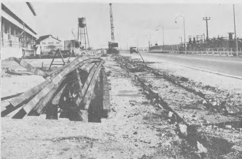
WITH THE aid of a ten-ton capacity crane, Mechanical-Yard riggers pulled old rails out of the asphalt like a dentist pulling a row of bad teeth. The track had to be removed from the area north of the main refinery road in the vicinity of Lago's general shops so that the road can be relocated. For many years, work trains such as the one pictured at left hauled general cargo throughout the refinery from dock-side unloading stations.
